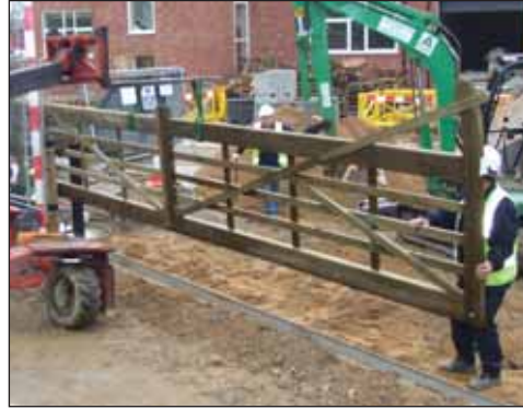
5 Bar Sliding Gate - Installation
